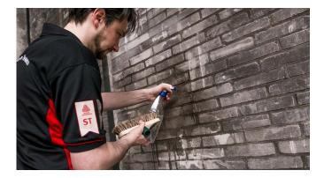
> Prior to applying the film the wall needs to be cleaned properly. Water, high pressure water cleaning devices or special cleaning fluids may be used, depending on the condition of the surface.
