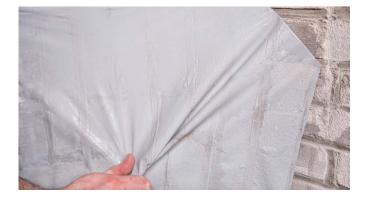
> For removal of the product, use the heat gun to achieve medium to high heat for best possible results. Remove the films slowly. Start at the top of the graphic and pull it from the wall at a 120-180 degree angle. Re-apply heat if required.
