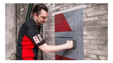
> Use a roller to apply pressure for the material to properly anchor to the surface and create a strong bond.
