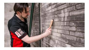
> On plastered or brick walls remove all dirt or other contaminants by use of a brush. It is recommended to brush the surface immediately before application to remove any dust or dirt that may have collected during the drying period.
