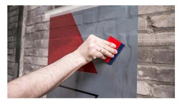
> Once fixated, pull the rest of the liner off the film and put the graphic into its final position. Apply light pressure with your hand or squeegee on the overall surface of the application, creating a light tack of the film onto the substrate.
