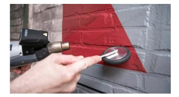
> For corrugated surfaces, use a heat gun and a small roller for a good finish. A temperature of up to 130°C with medium air flow setting may be used to soften the film. With the help of the roller, push the film into the textured surface of the wall. In case of application on a brick wall, start with the flat surface of the bricks first.
