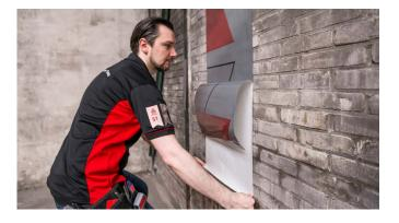
> Use two hands when pulling the liner from the film, using care not to stretch the film. Delaminate a few centimeter of the liner from the face film and fixate it at one corner of the application. For ease of application, the liner should be removed as close to the surface as possible.
